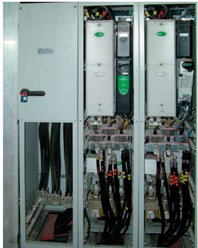
Pictured: SP9 with user designed incomer (interconnection made with SP P06 busbar kit)
