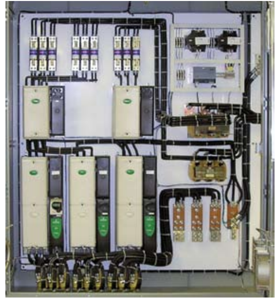
UL1, Ventilated Encl., SPM, 600 hp, 460VAC
